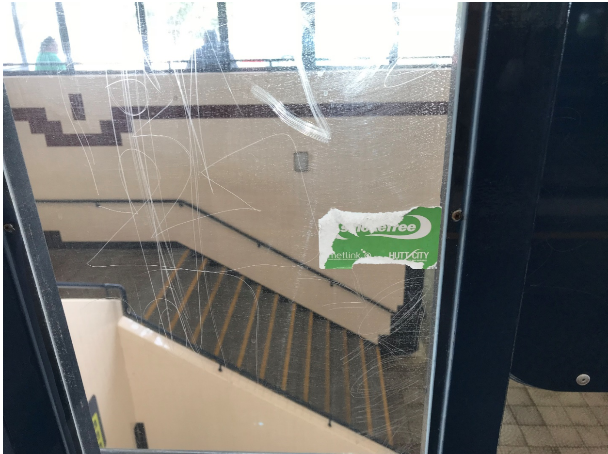
Figure A9: Smokefree sticker sign showing evidence of vandalism (Waterloo railway station, Lower Hutt). Of note is that such stickers appear to be frequently subject to such vandalism.
