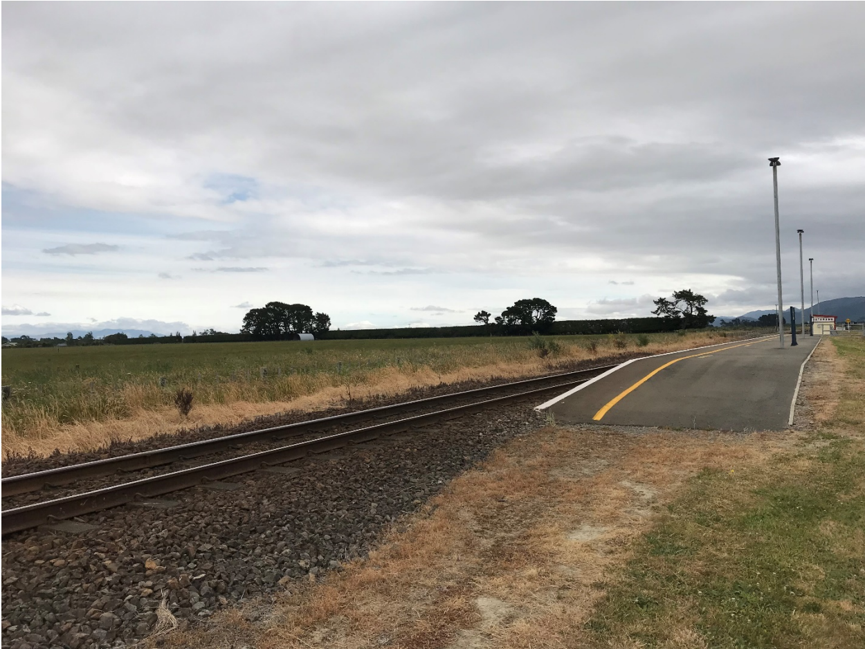
Figure A1: Railway platform in a remote rural area which also shows a large grassed area over which pedestrians could easily traverse and which we defined as an “entrance area” (Matarawa railway station, Wairarapa).
