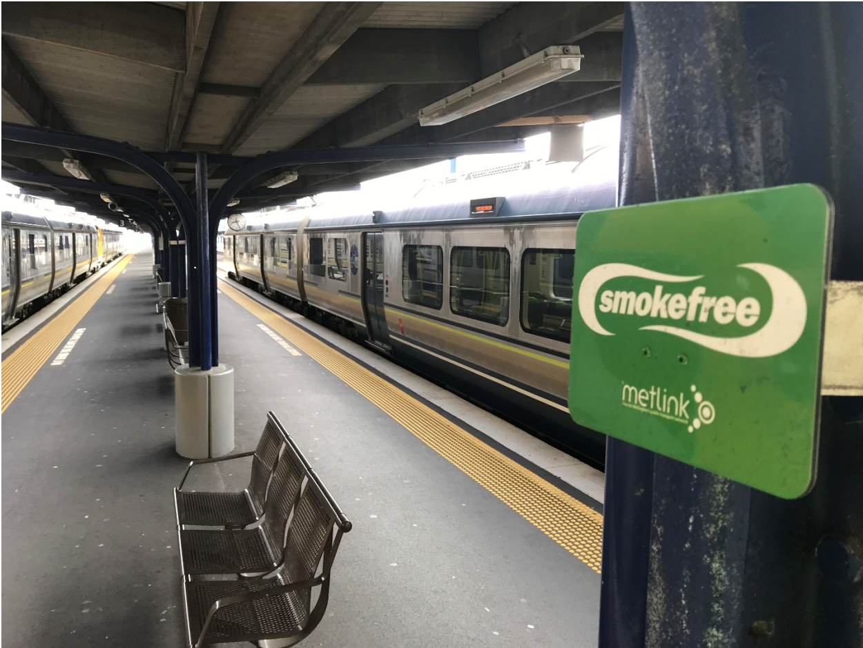
Figure A8: Common smokefree signs on many of the supporting posts on Wellington main railway station platforms (n = 164 such signs at this station).
